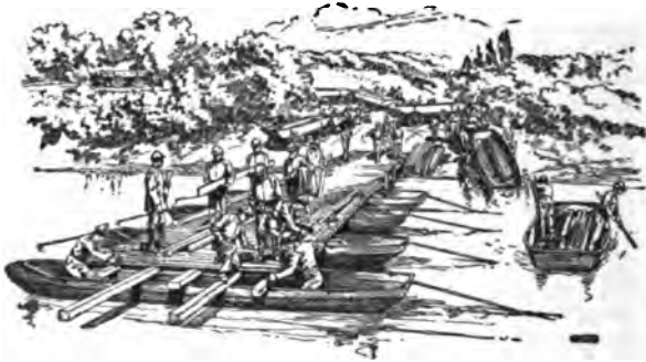
BUILDING A PONTOON BRIDGE.
